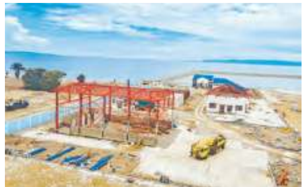
KAREMA Port, a new container terminal, on the verge of completion.
