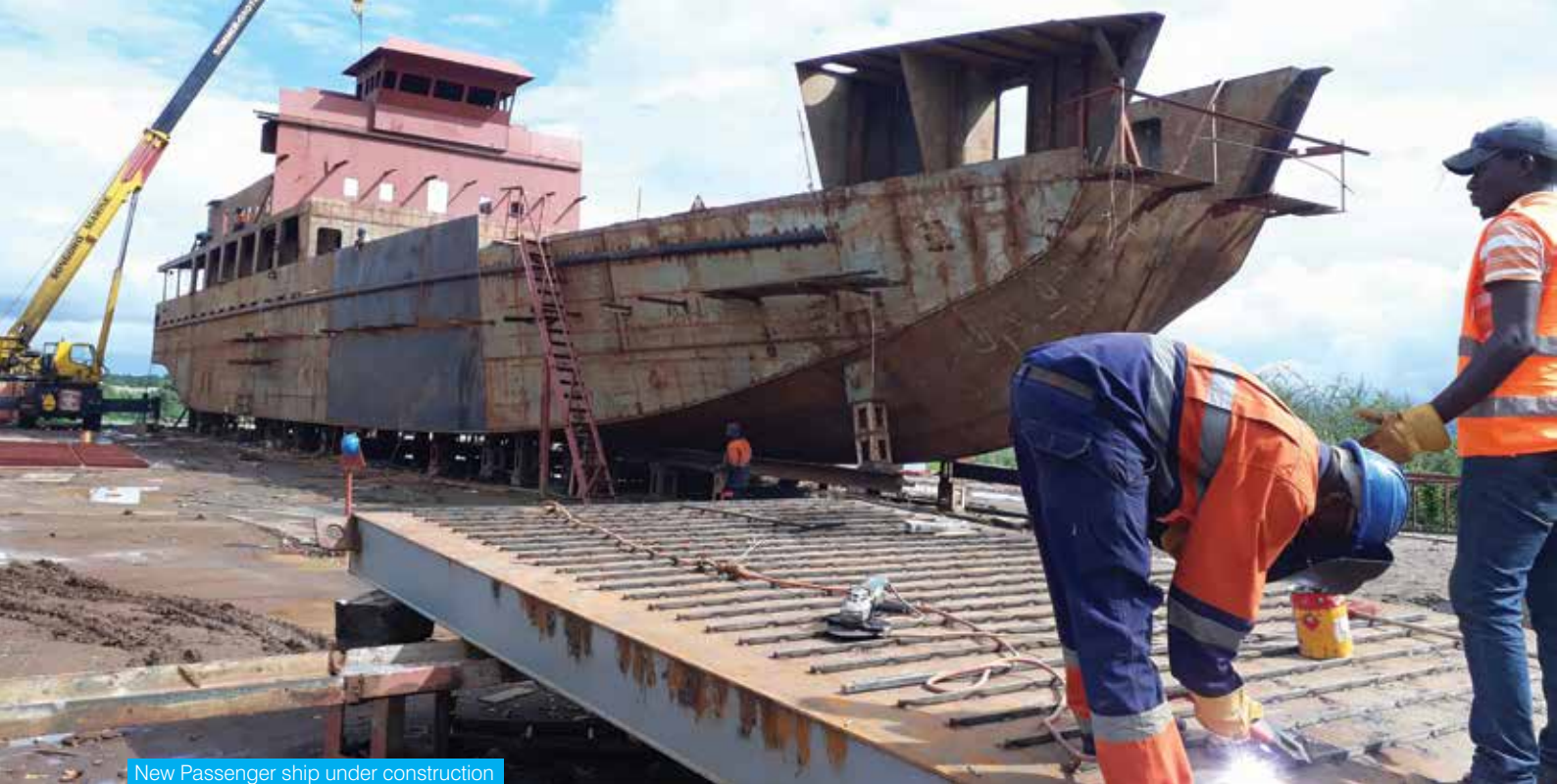
New Passenger ship under construction
